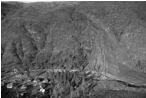
Figure 17: Coastal mudslide on Highway 50, California following vegetation removal and heavy rainfall. Source: Eplett, R.A., California Governor's Office of Emergency Services.
