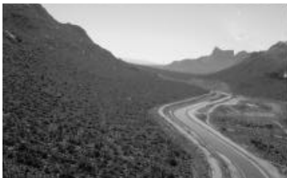
Figure 1: The Central Arizona Project brings Colorado River water 330 miles uphill to Tucson and Phoenix, Arizona. Source: K. Jacobs
