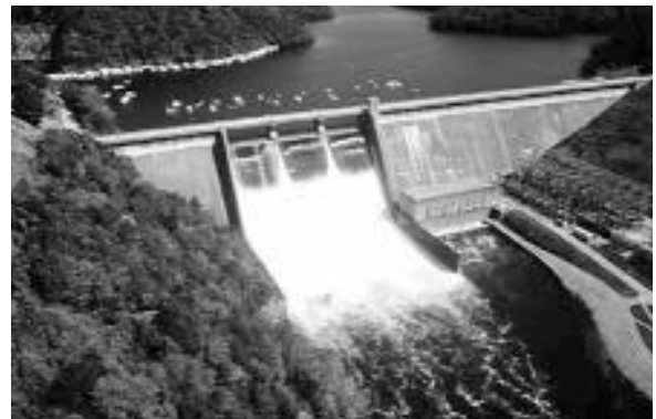
Figure 3: TVA has more than 50 dams in seven states. Source: Tennessee Valley Authority
