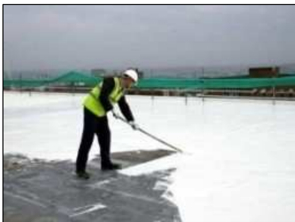
Figure 3: Creating a white roof is relatively simple
