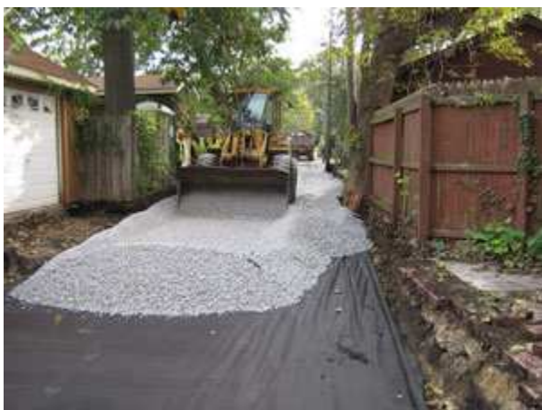
Figure 6: A green alley is installed in Chicago
