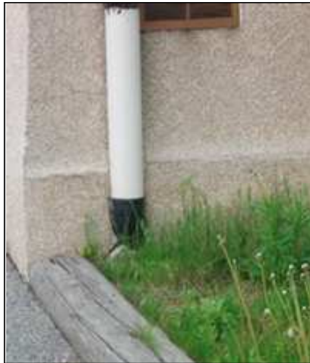
Figure 5: (Left) A gutter downspout connected to the storm drain system. (Right) A disconnected downspout using a rain barrel to collect stormwater for a rain garden
