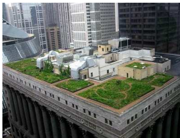
Figure 2: Chicago's City Hall Green Roof
