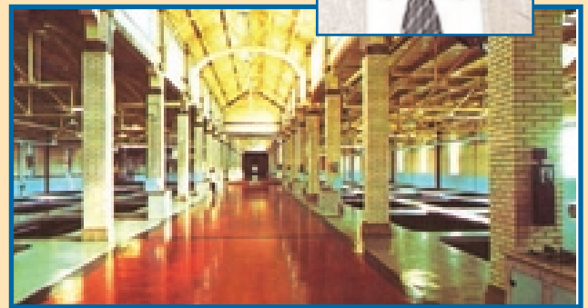
This Minneapolis Water Works treatment facility is part of the utility's $1 billion distribution infrastructure system.
