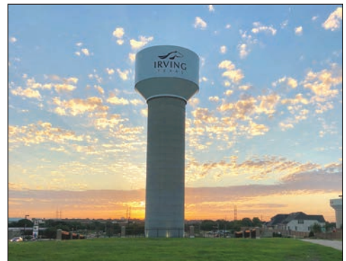
TOP: The under-construction Northgate Ground Storage Tank is planned for completion in late 2022.
