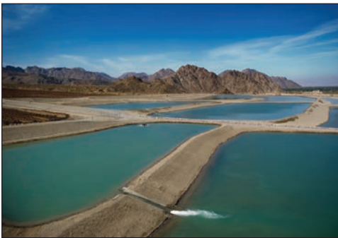
TOP: Whitewater River Groundwater Replenishment Facility
