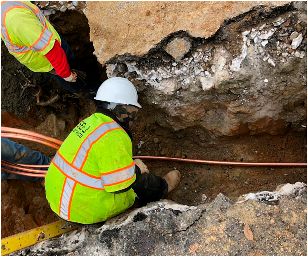
DC Water professionals remove lead service lines.
