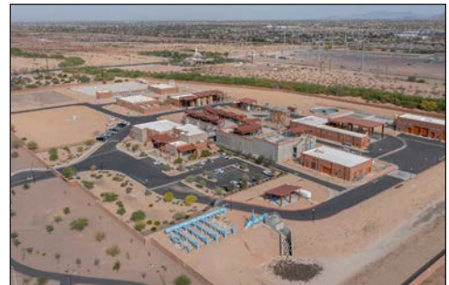
TOP: The Central Arizona Project and Brown Road Water Treatment Plant are pictured. The Department works to effectively manage its supply of Colorado River water through a variety of means.
