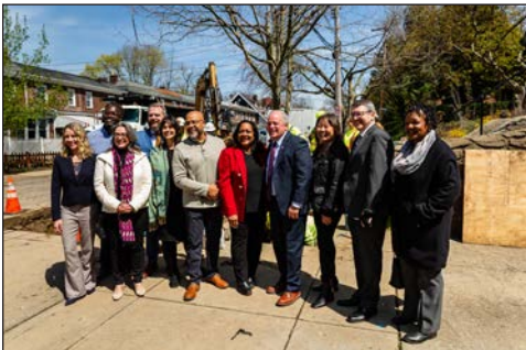
TOP: Local leaders, PWSA staff, and media gather as PWSA contractors replace its 10,000th lead service line in the Hazelwood neighborhood of Pittsburgh in February 2023.
