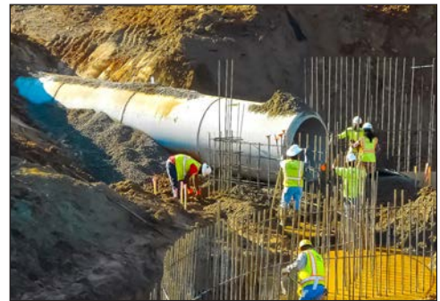
TOP: Cook Park work site
