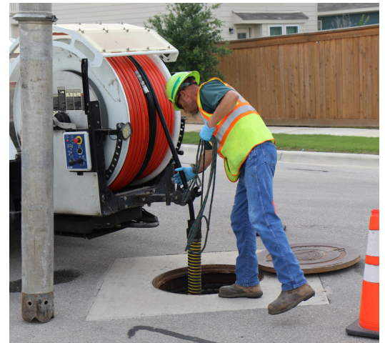
TOP: Crew members work to uncover a leak on an 8-inch water main.
