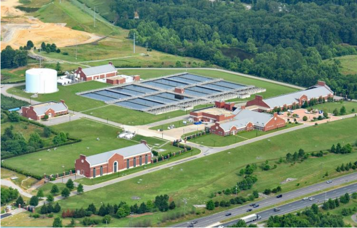
Griffith Water Treatment Plant
