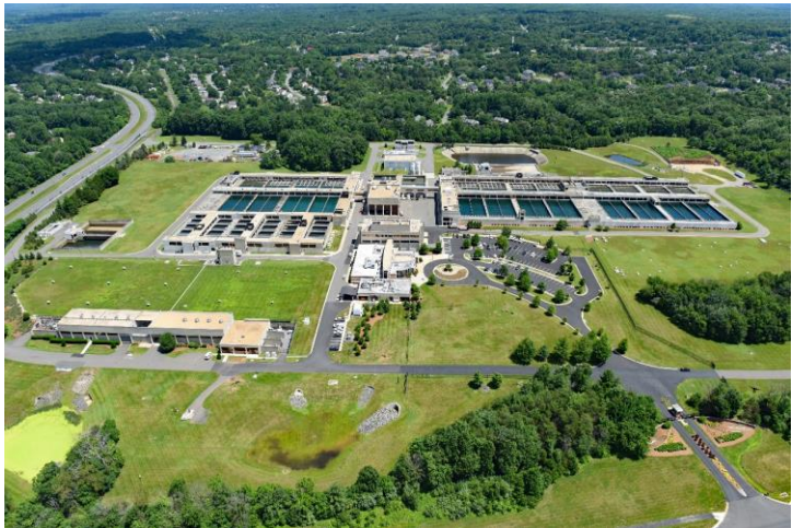
Corbalis Water Treatment Plant
