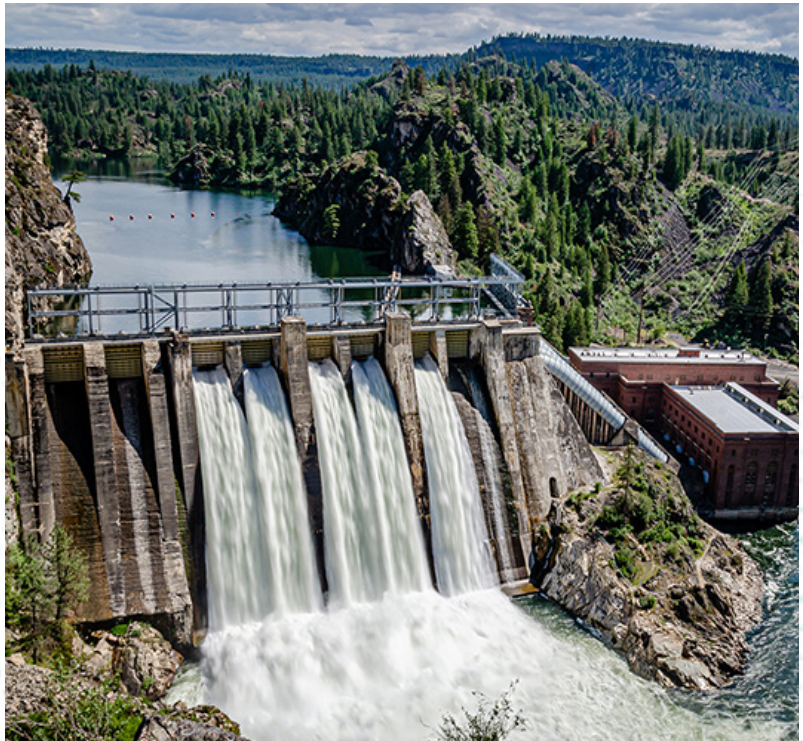
Above: Long Lake Dam on the Spokane River
