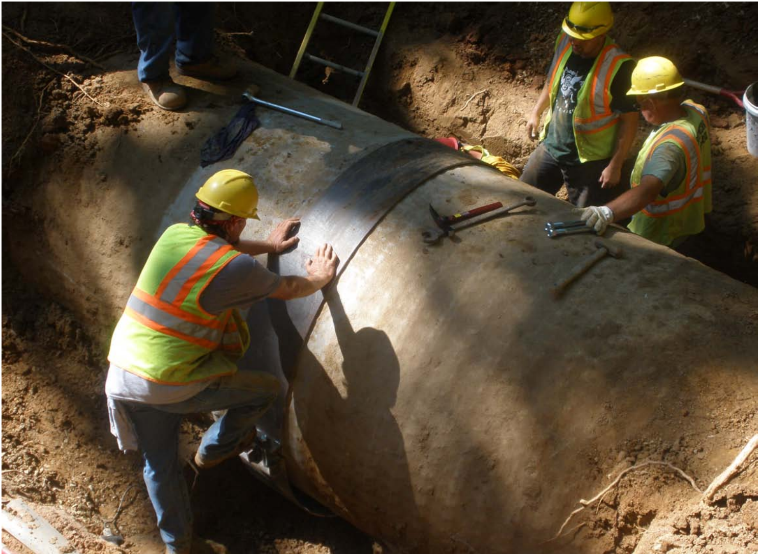
The use of steel bands,
