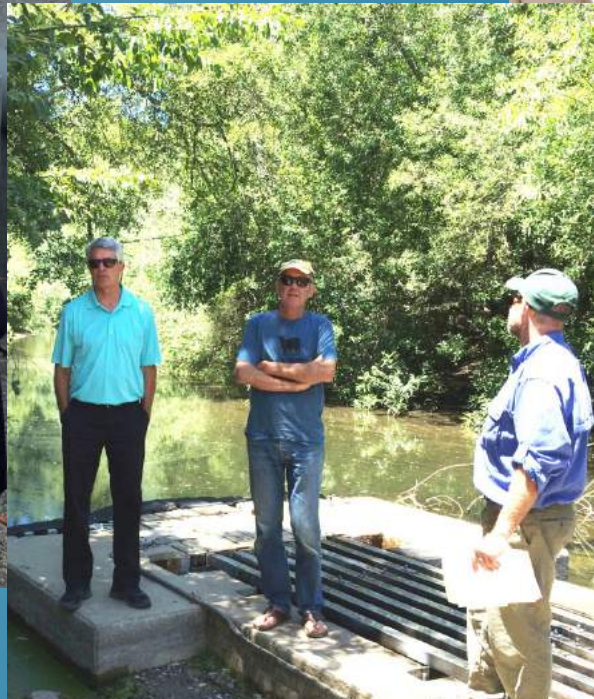
River intake (drought conditions)
