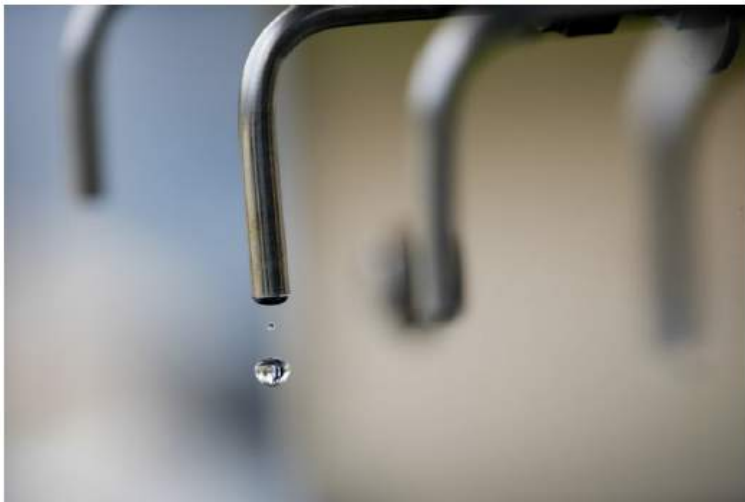
A test spout on a reverse osmosis container at San Diego's Advanced Water Purification Facility (AP Photo/Gregory Bull)
