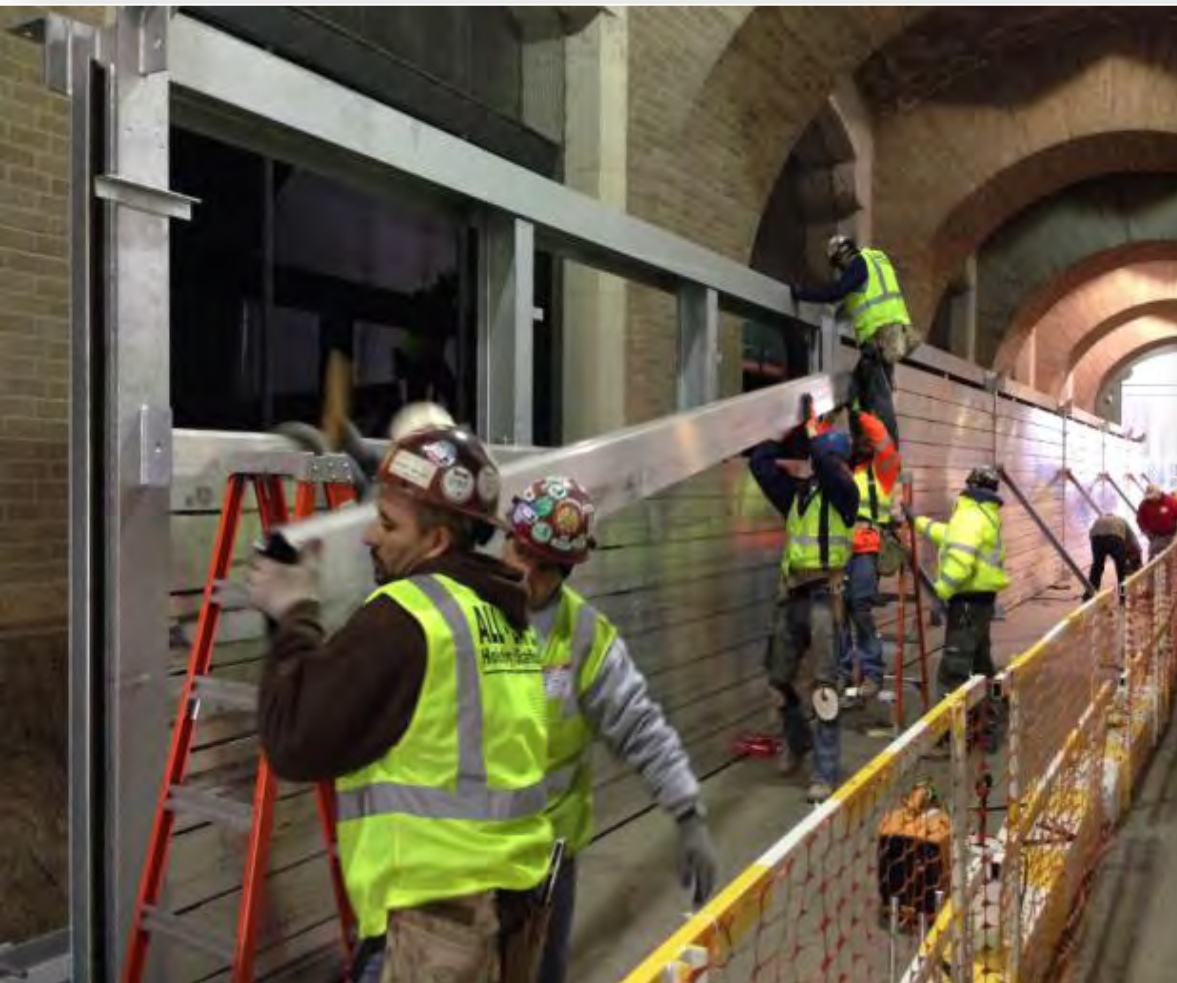
Images: deployment of removable flood wall - flood wall design – underground utilities and conduit plugs
