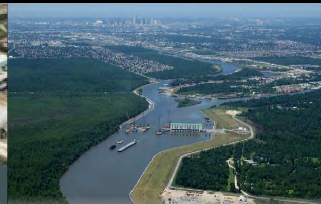
West Closure – Pump Station
