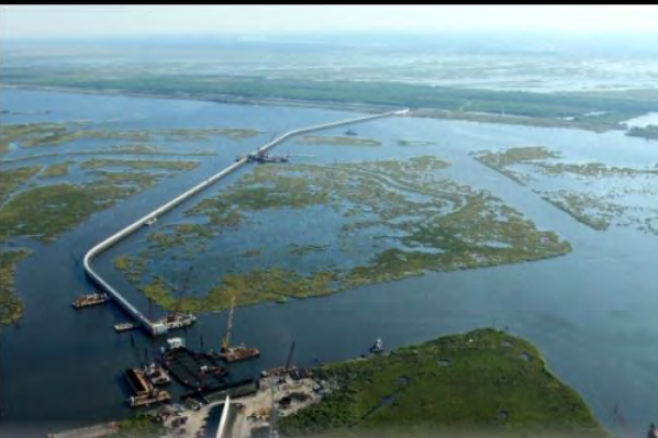
Lake Borgne Storm Surge Barrier
