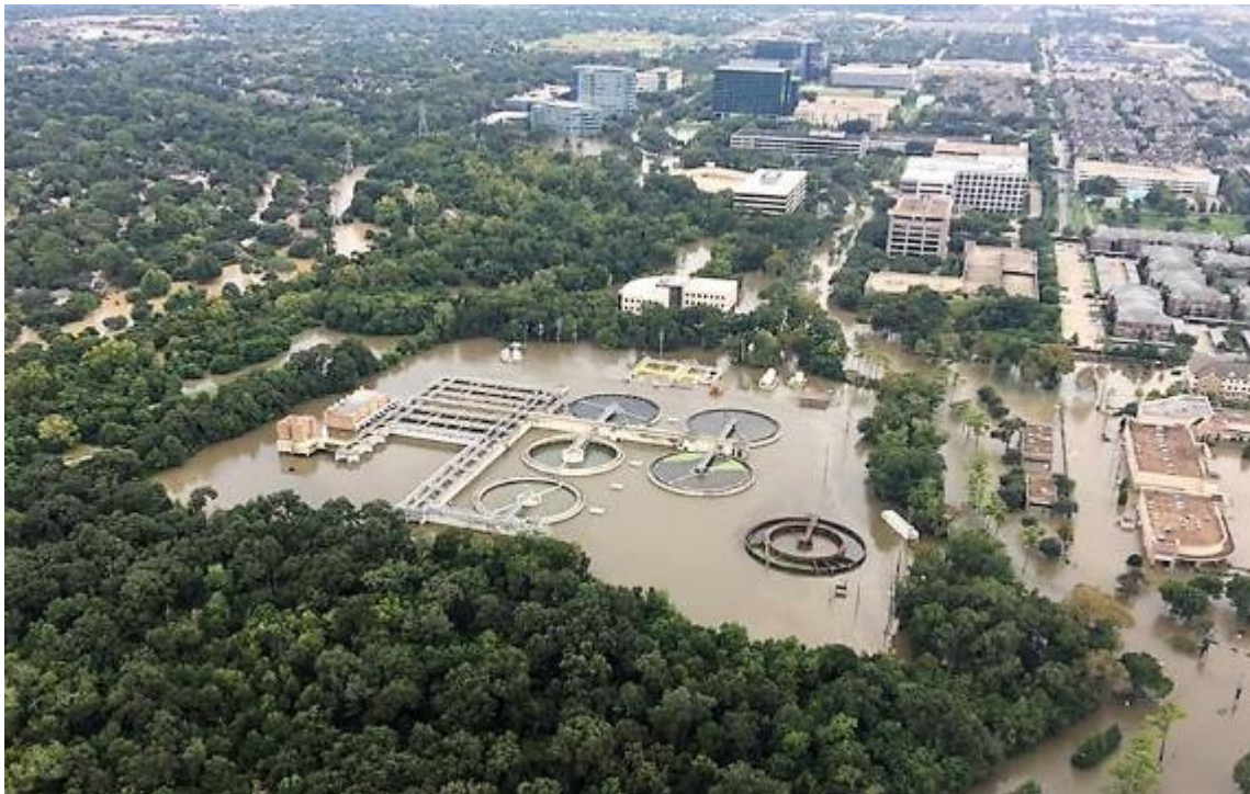
Turkey Creek Wastewater Treatment Plant
