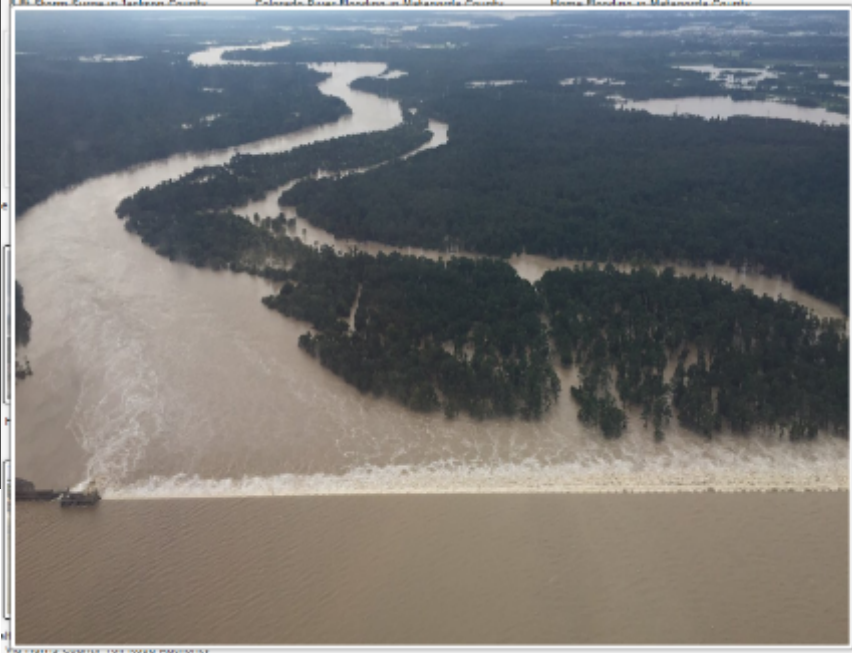
Lake Houston Spillway 8/30/17
